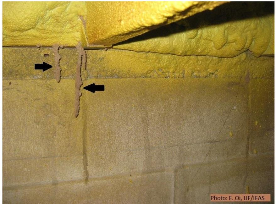
Figure 1 Subterranean Termite tubes emerging from behind spray foam insulation installed over floor joists in a crawl space.
